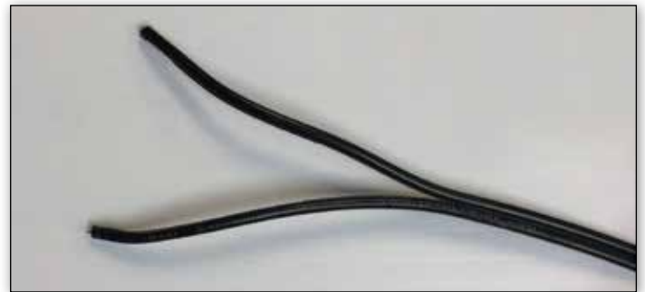
2 Conductor Wires running to basement 12V Power Transformer
